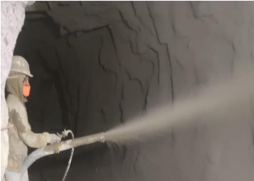
Photo: Tunnel shotcrete works during construction
